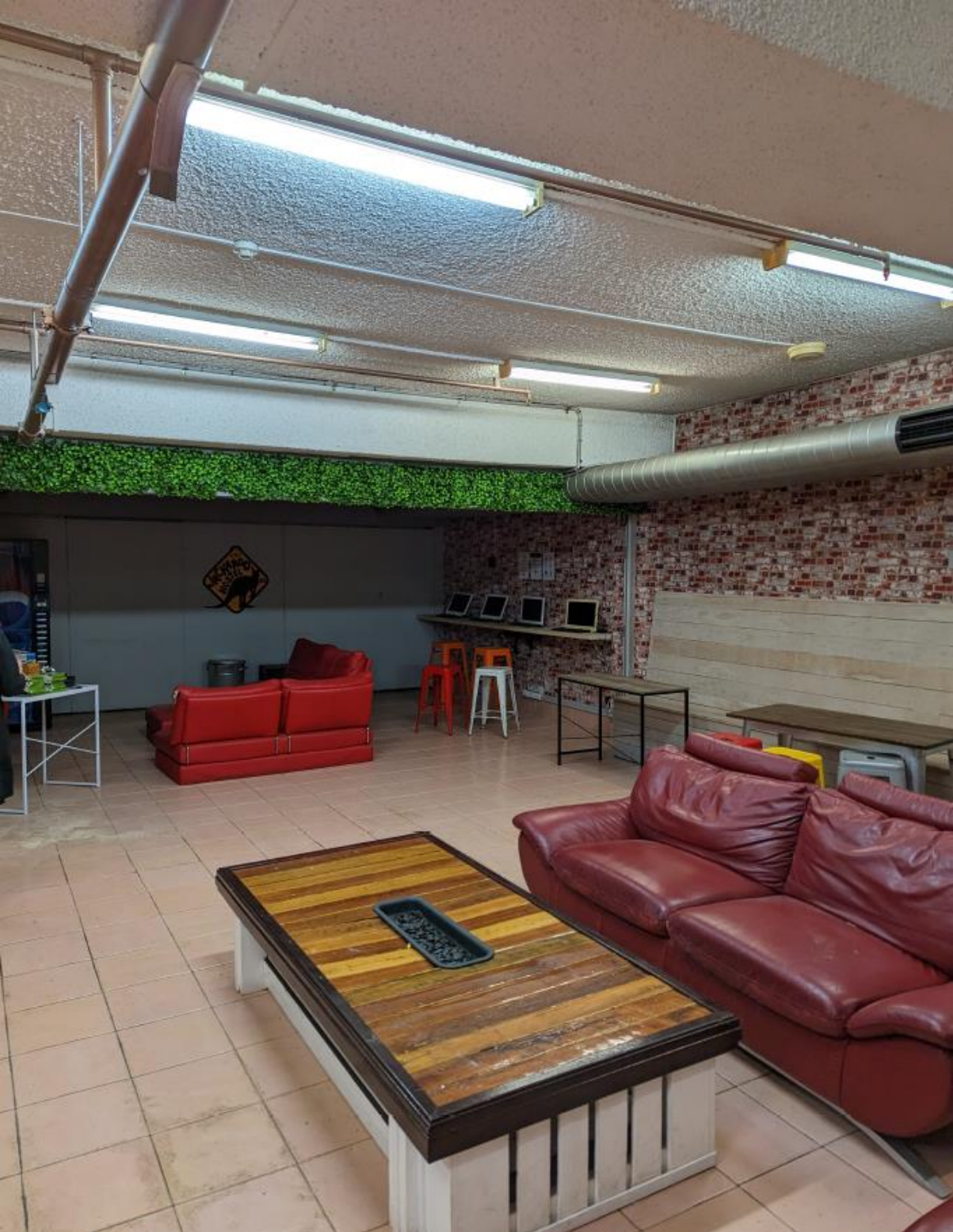
Figure 7: Existing basement level 1
