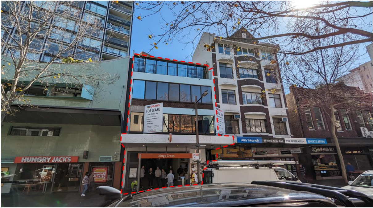
Figure 2: Front of the site viewed from Darlinghurst Road, looking west
