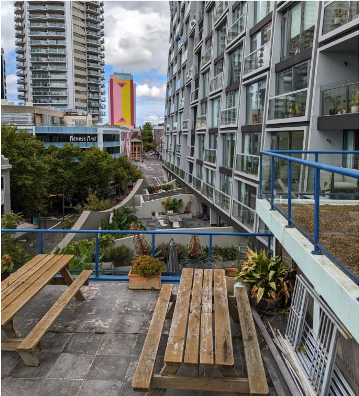
Figure 15: Eastern side of existing rooftop terrace at the front of the building looking south
