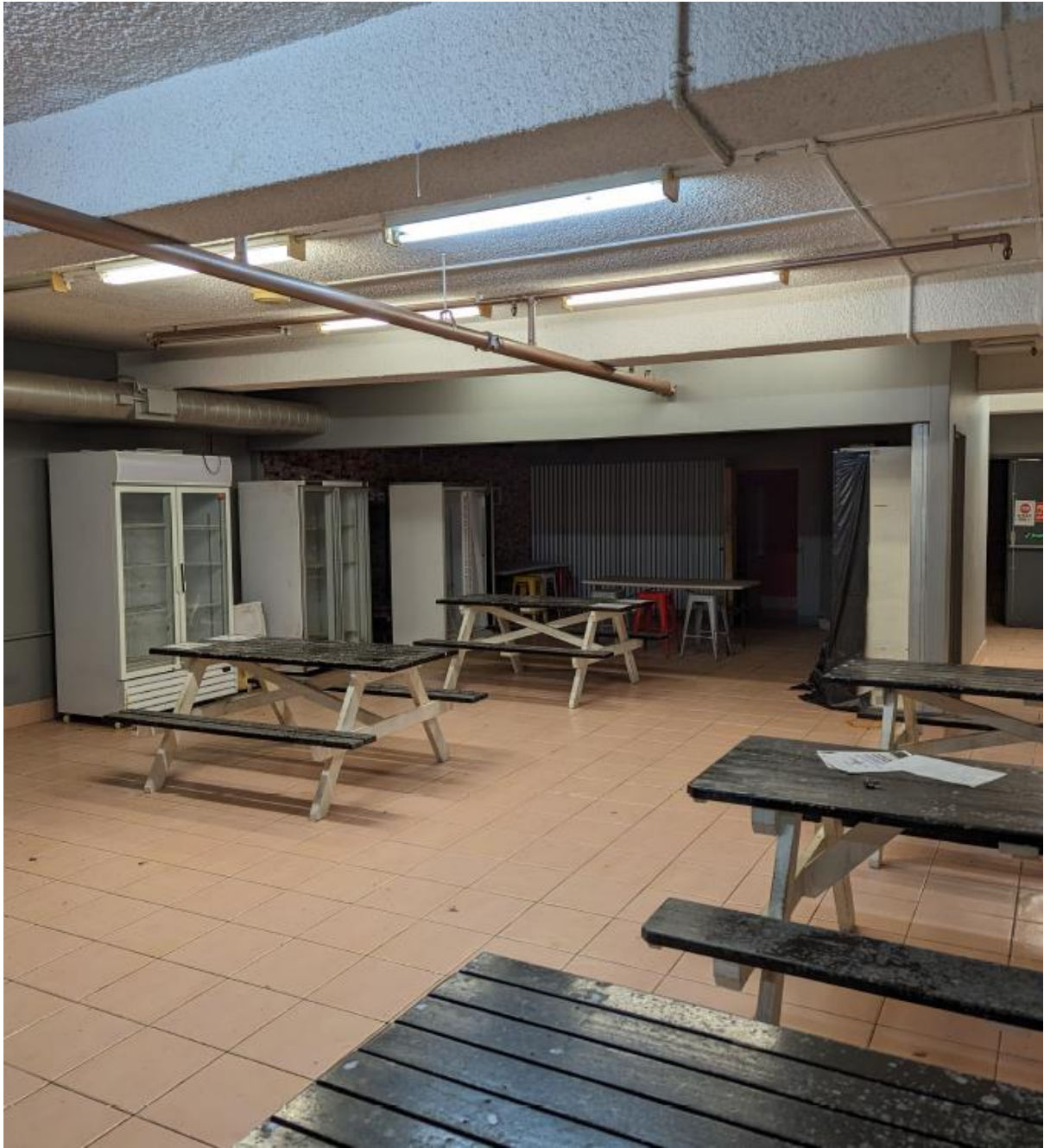
Figure 6: Existing basement level 2
